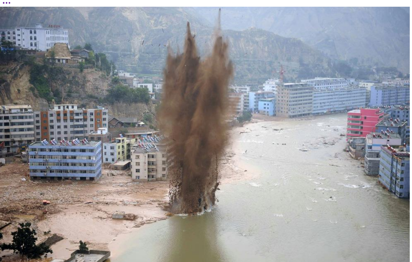
Chinese rescuers use explosives in an attempt to clear blockages and release the water of Bailong River in Zhouqu, China on August 11, 2010. (STR/AFP/Getty Images)
