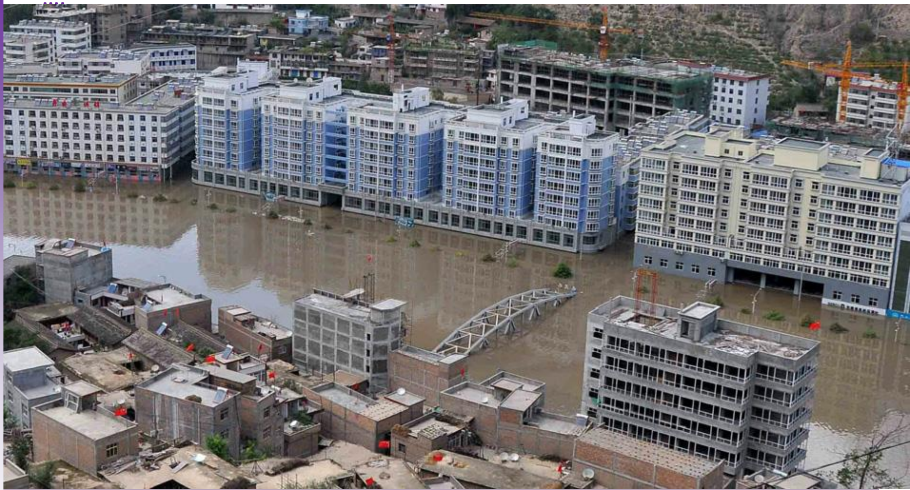
Aerial view of the flooding in Zhouqu county. (STR/AFP/Getty Images)
